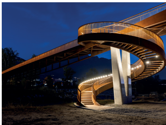
LaneLED WALL, Passerella Torretta Bellinzona
